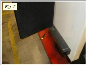
CAUTION-- Before you begin the adjustment, take the precaution of securing the top frame. It will be necessary to lift up on the speaker frame as you make this adjustment. This could result in the top frame coming loose from the wall. Painter's tape can help to prevent the top frame from being pushed upward during the speaker angle adjustment.
